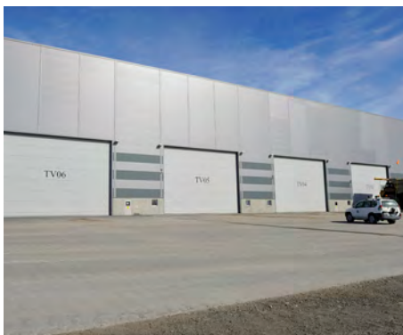
Truck workshop with associated wash bay and tire workshop.
